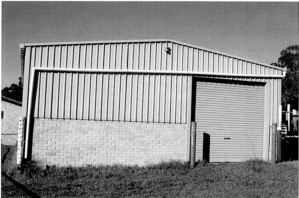
Photo 6 – View of the northern wall of the garage to the south.
