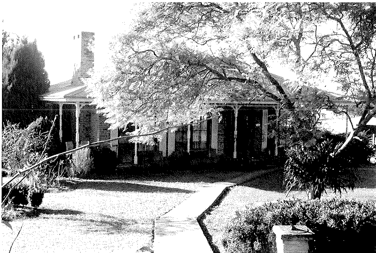
Photo 1 – View from the west to the east of the main residence.
