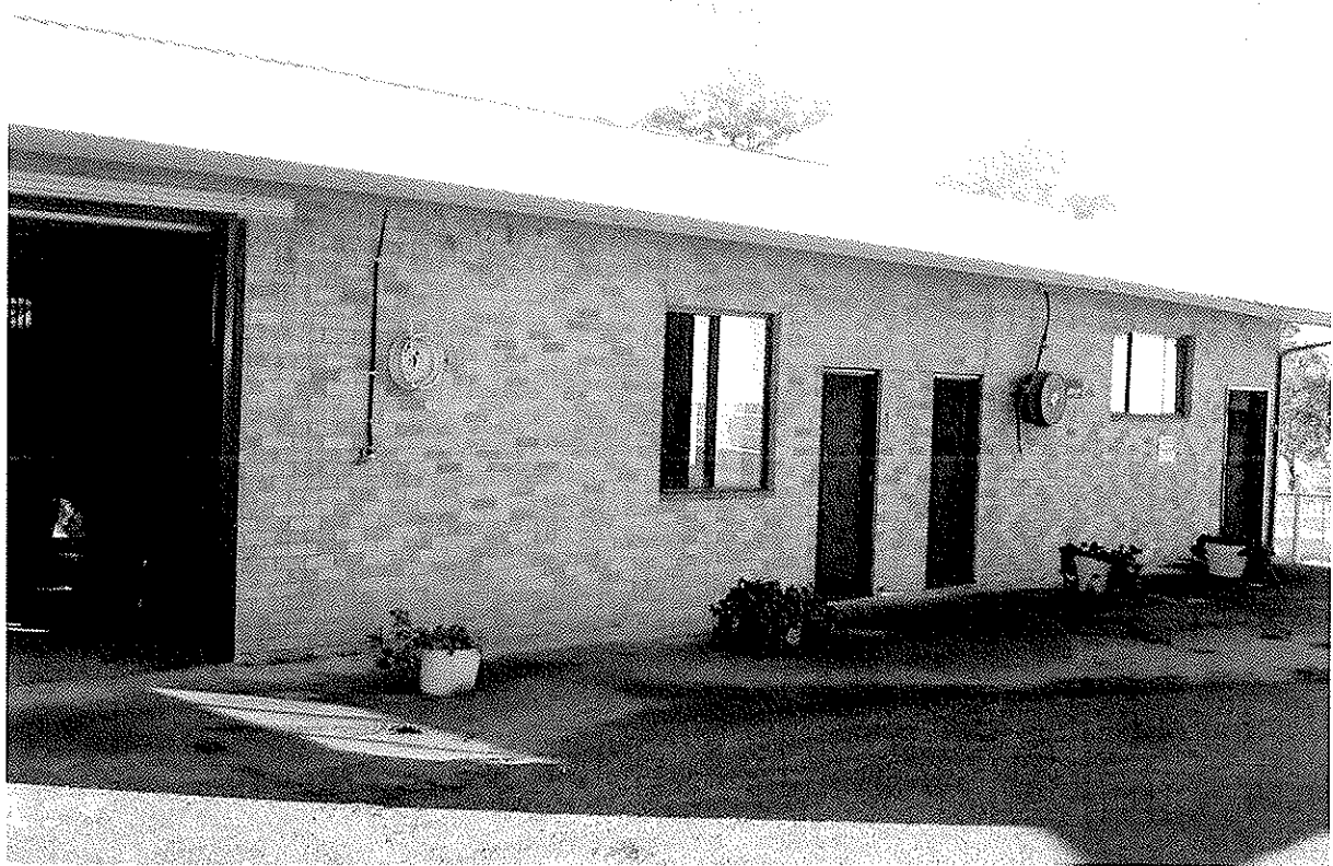
Photo 7 – View of the western wall of "The Cottage" to the south-east.
