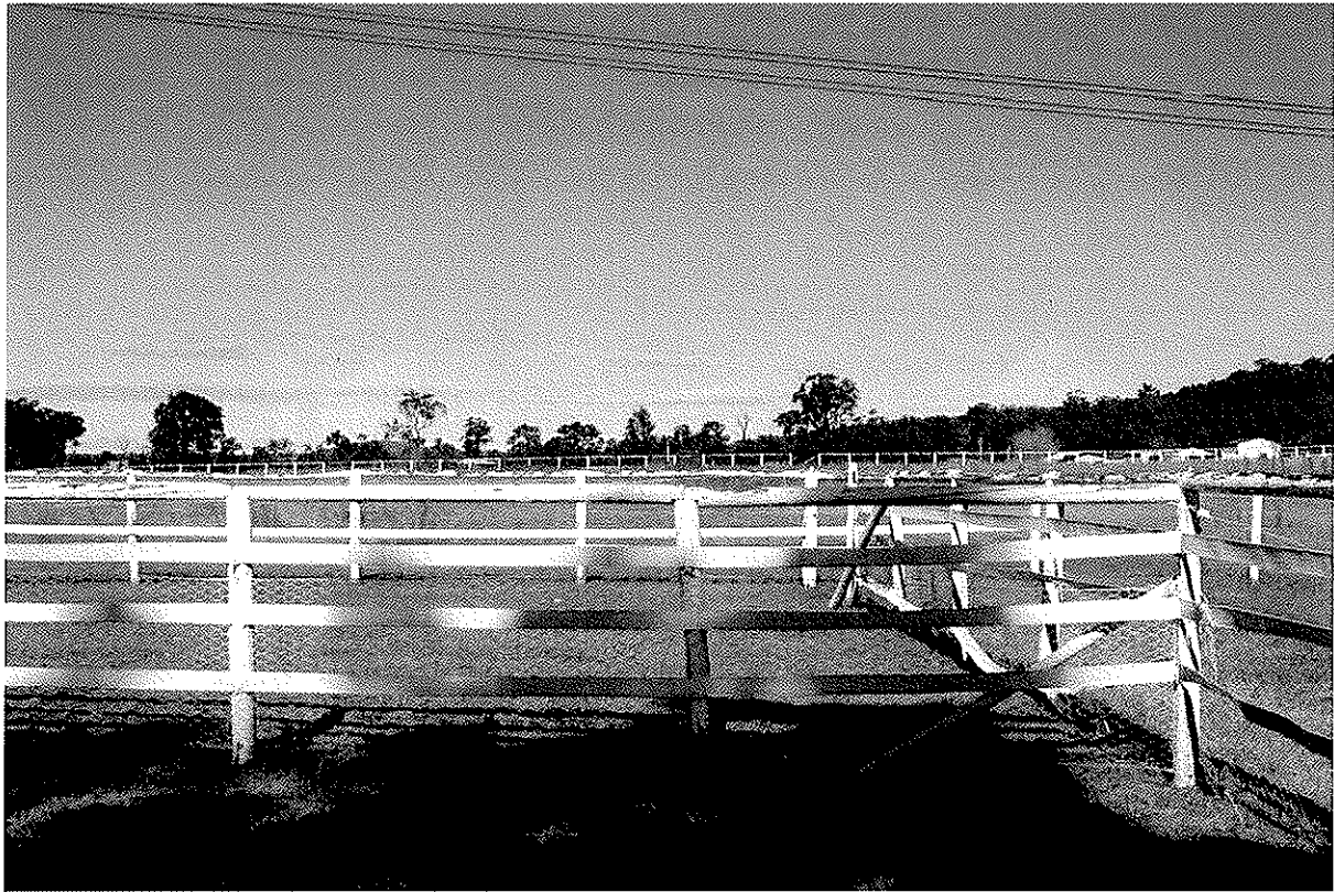
Photo 21 – View to the south of paddock fencing across the northern portion of the site.
