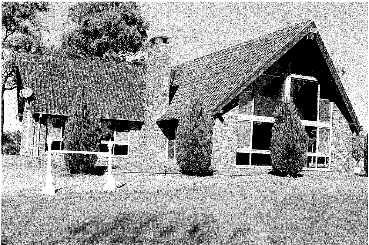
Photo 14 – View to the south-west of the vacant residence located in the south-eastern portion of the site.
